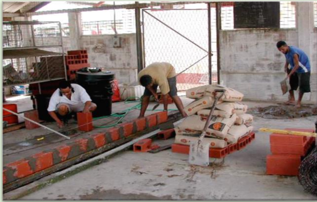
Graduate students building the concrete floor pens
